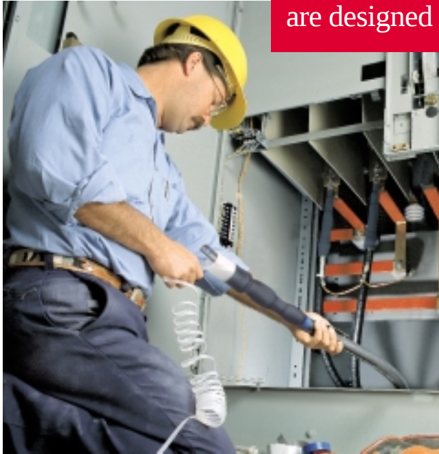
Cold Shrink QT-III Indoor Termination
